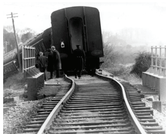
Example of a railway bridge strike.
